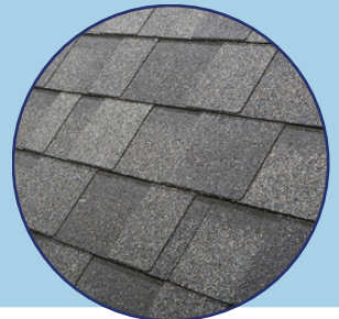
SHINGLES / TORCH-ON ROOFING
